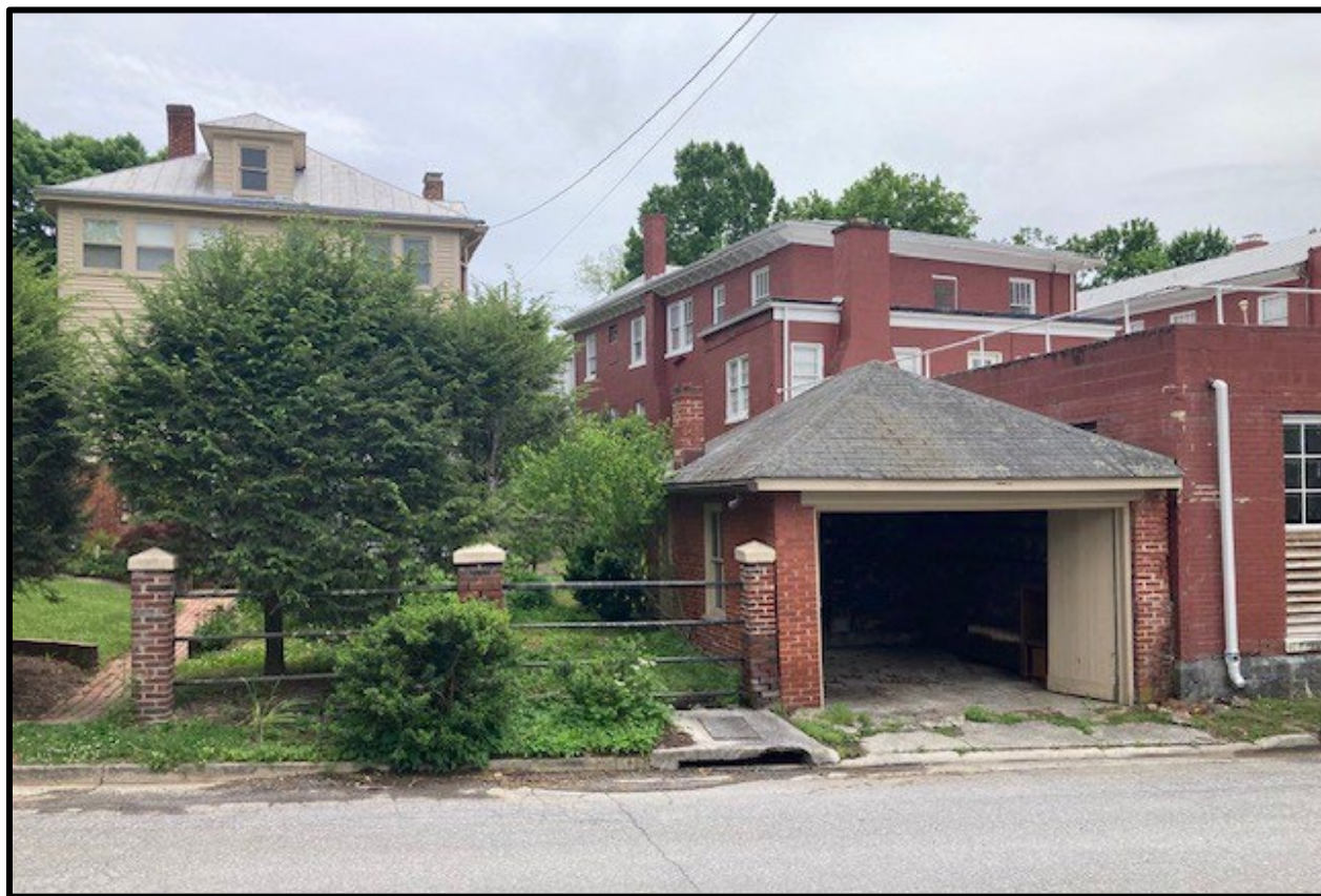
405 S. Main Street garage existing conditions
