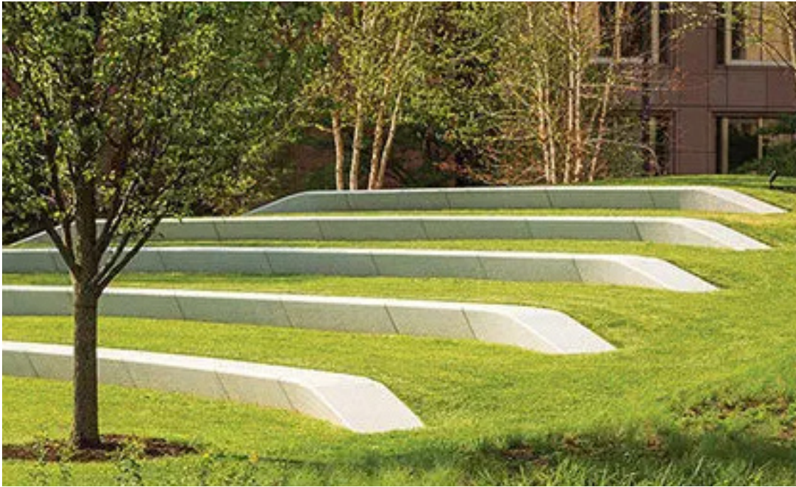
Concrete Seat Wall
