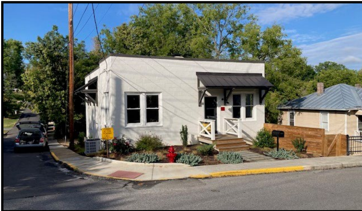
View of subject parcel from Diamond Street
