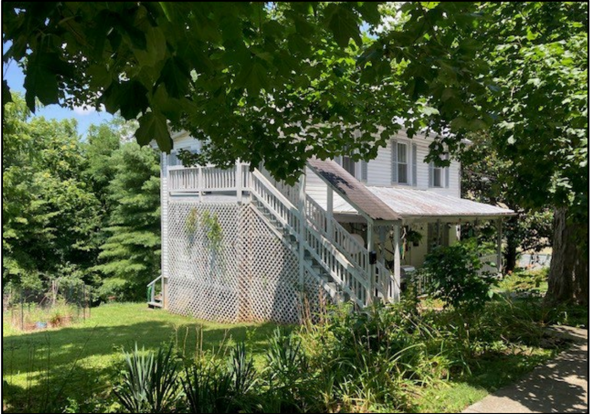
photographs of 10 N. Lewis Street
