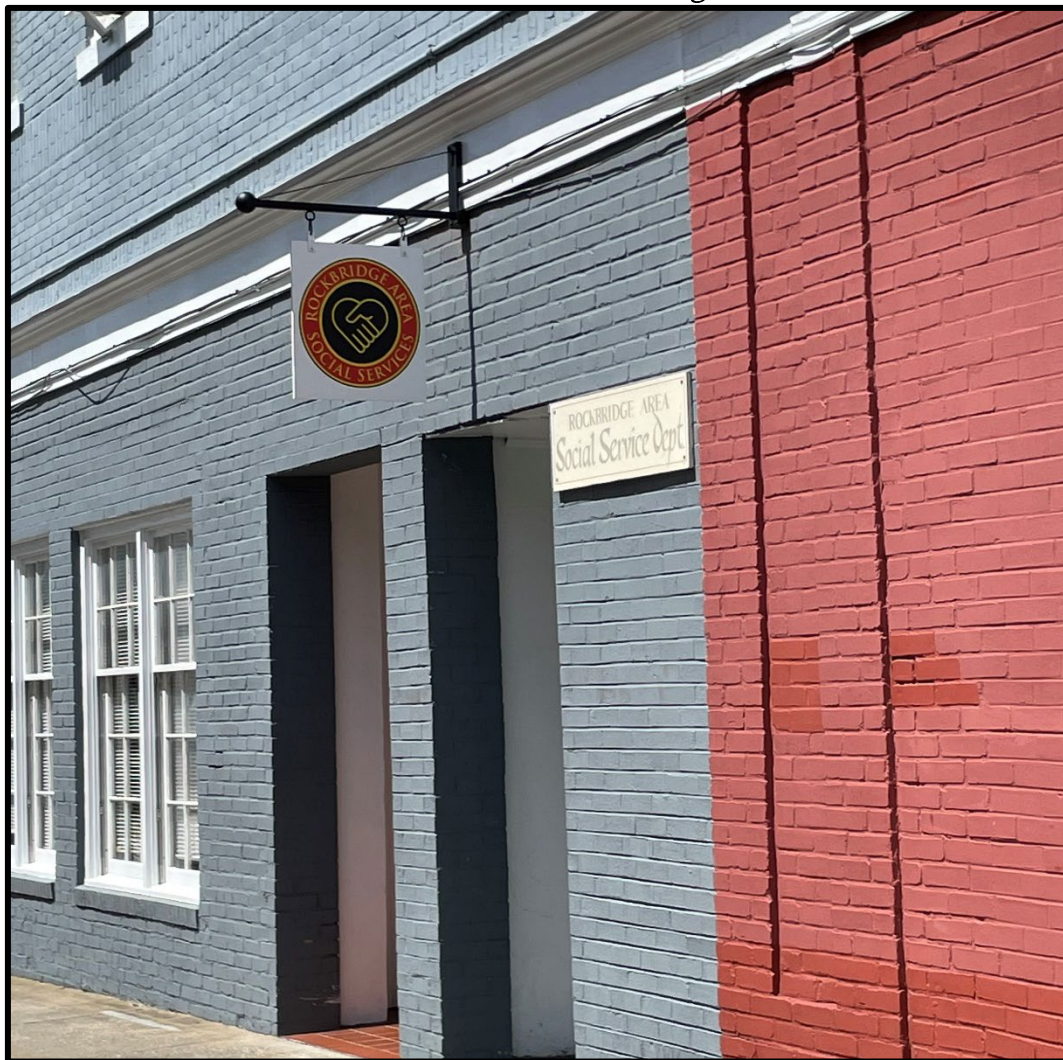
20 East Preston Street existing conditions
