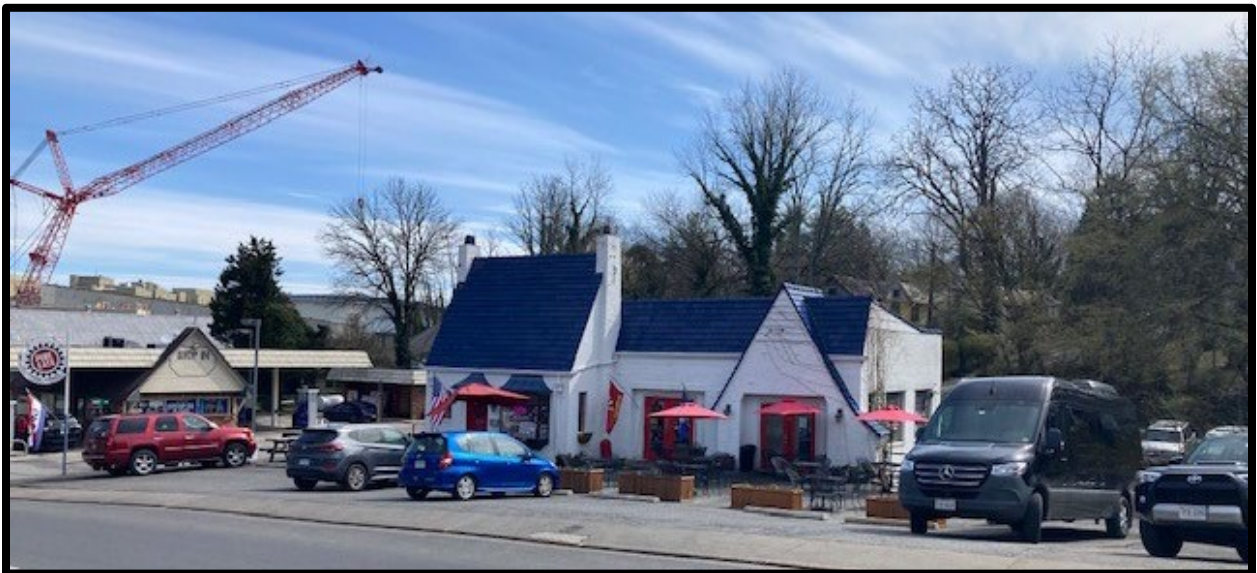
photograph of existing conditions 107 North Main Street
