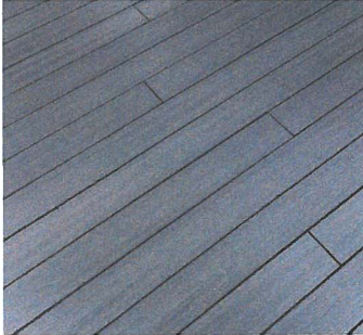
T & G Wood Decking, Painted
