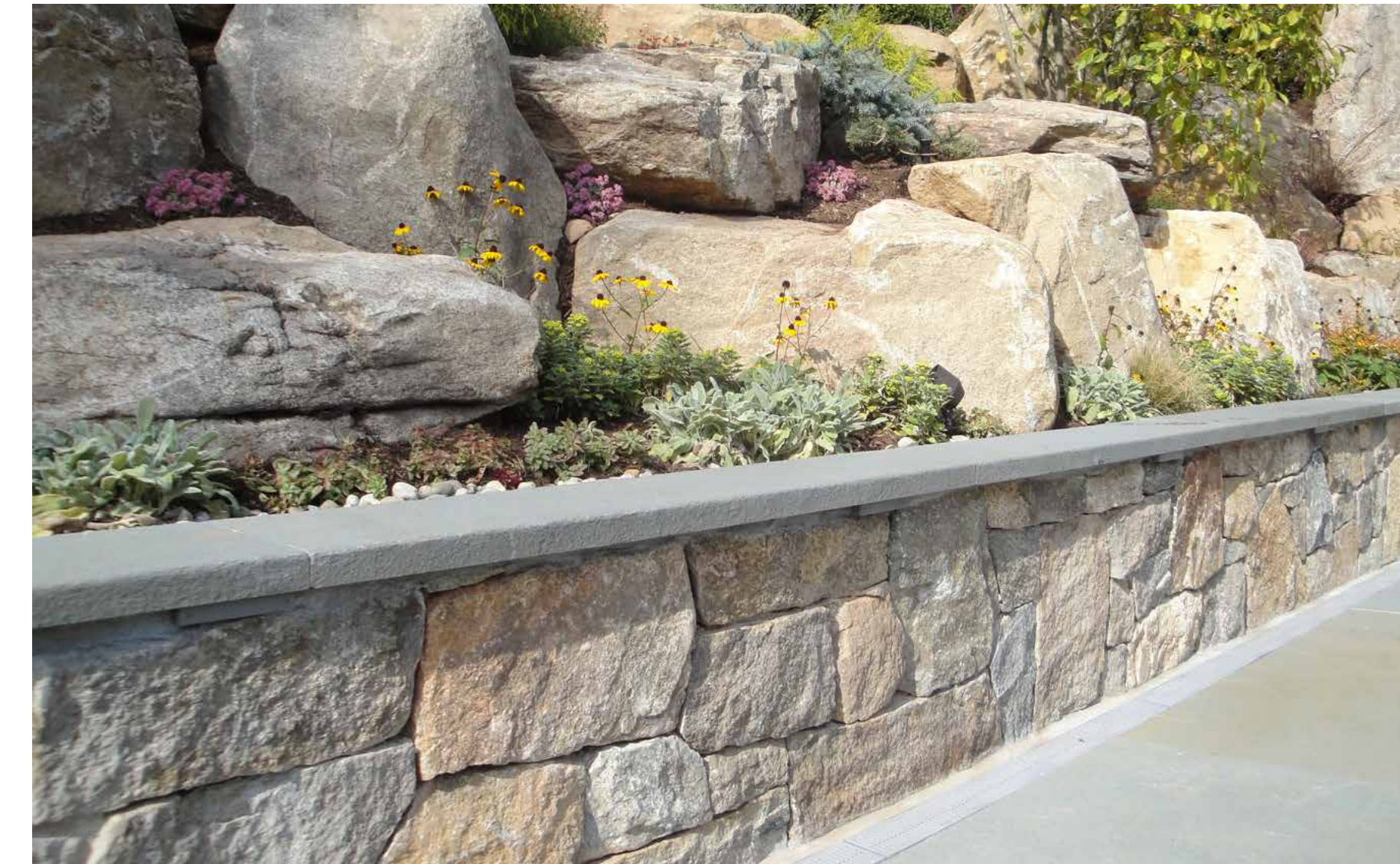
H. Seat wall at sign plaza.
