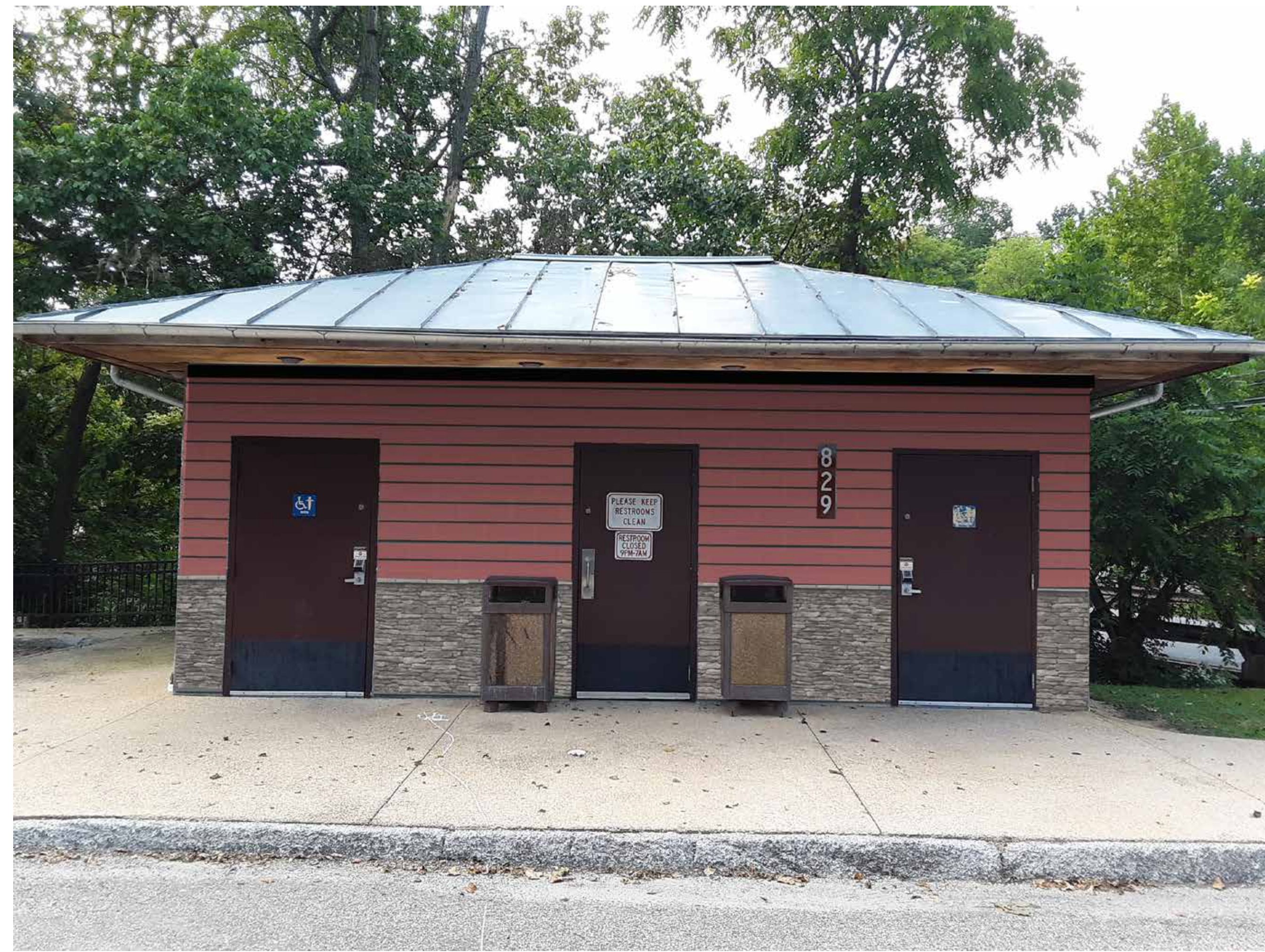
EE. After: Cladding on restroom facade, compatible with the Miller House
