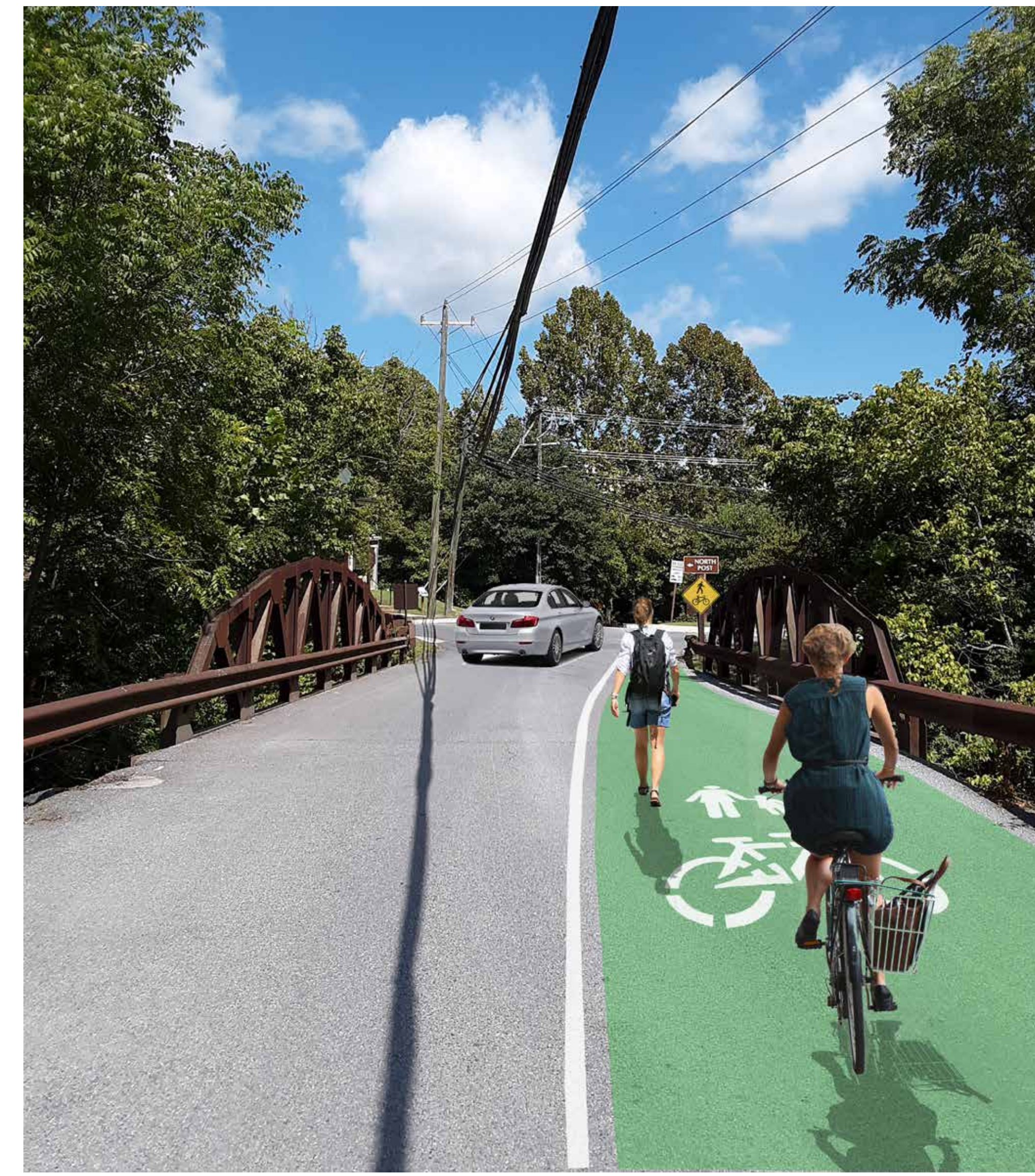
N. After: Bridge at Park Entrance with a one-way 14' driving lane and 8' bike/ped path
