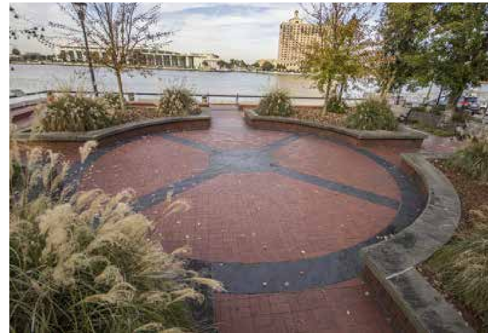
E. Sign Plaza - highlights the convergence of several walkways and entrance to the overlook. Historic signs may be integrated into the space with seat walls for pausing.
